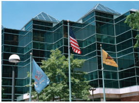
Downtown Milwaukee Campus 700 West State Street Milwaukee, WI 53233
