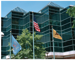
Downtown Milwaukee Campus 700 West State Street Milwaukee, WI 53233
